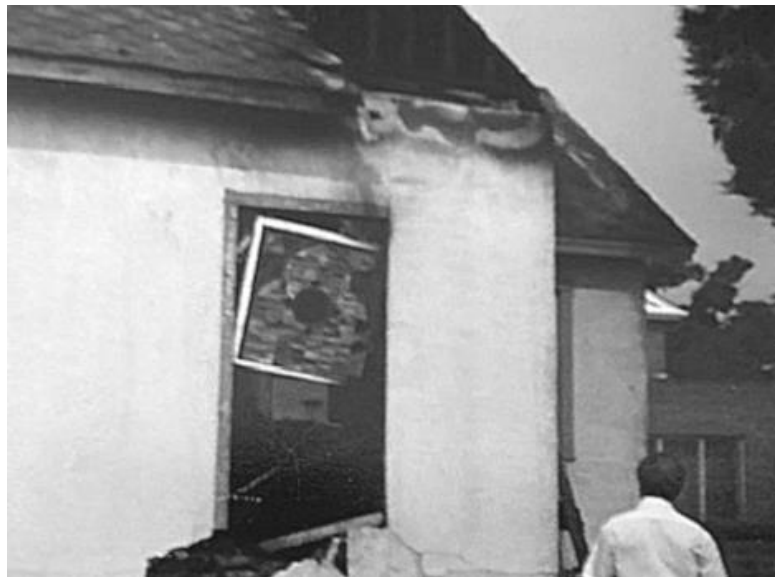
Inspecting the exterior damage, including one of the memorial windows that were destroyed
