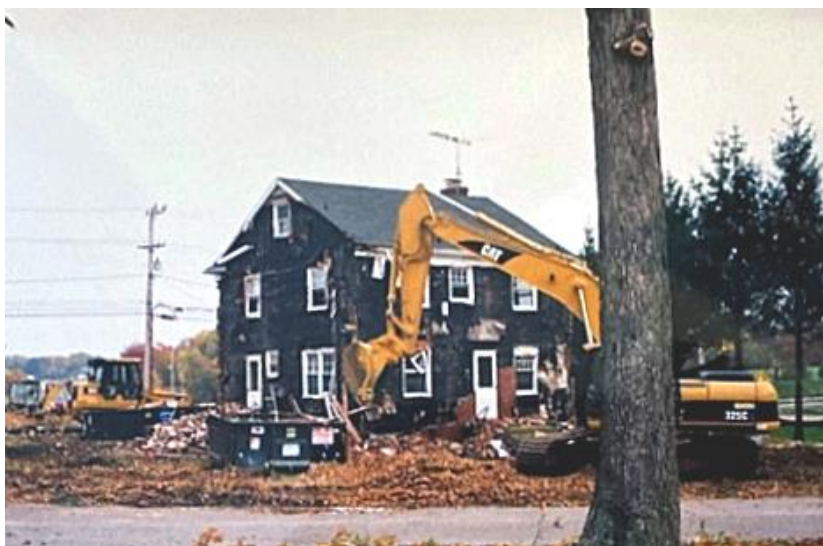
The Camp Chapel Parsonage during its demolition.
